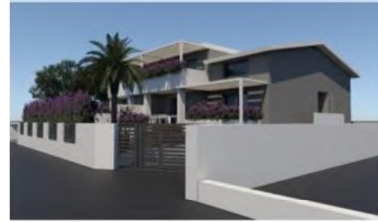
Monza MB - 2021 Private residence arch. Francesco Aiello arch. Davide Tresoldi Semi-detached house.
