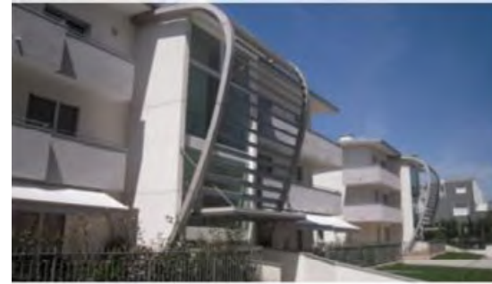
Seregno MB — 2009 Residential compier 5420 sqm arch. .2soldi co-progettista arch.th A. A .nphi, R. Galliani The residential complex is divided into three blocks characterized by a round covering coated in aluminium. The drainpipes are inserted into the round beams that reach the ground by drawing a perfect continuation of covering. The stairwells are screened with a microperforated meta sunshade.
